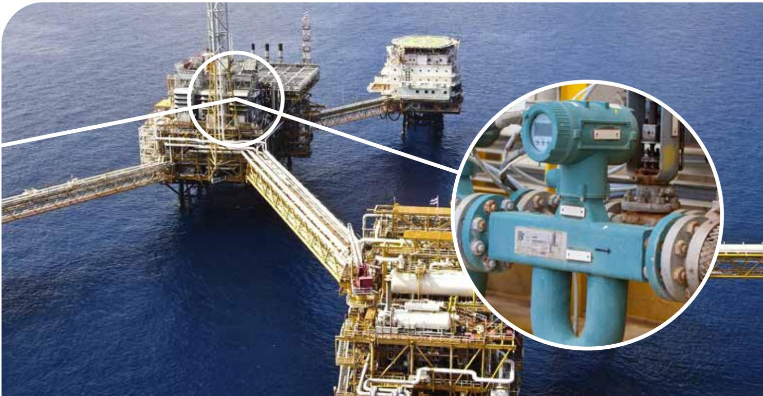
The use of Coriolis flow meters has become increasingly commonplace in the offshore oil and gas industry, as they are one of the most reliable instruments with which to determine flow measurement.
